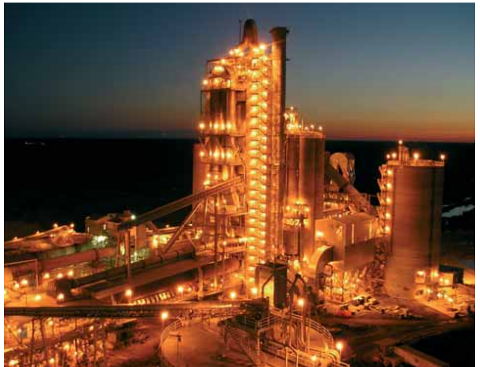
Harleyville cement factory. South Carolina. USA
