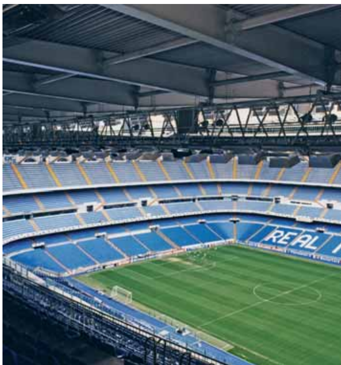
East roof on Santiago Bernabeu Stadium. Madrid
