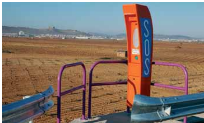
Upkeep of the Los Viñedos dual carriageway. Castilla-La Mancha
