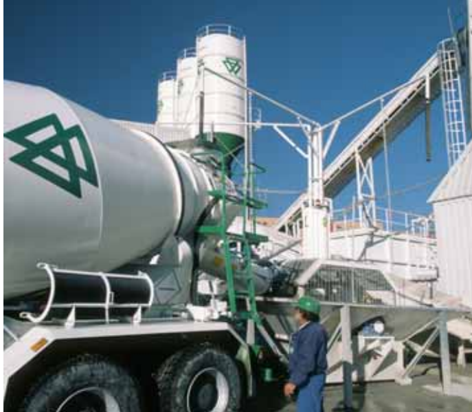
Hympsa concrete plant in Vicálvaro. Madrid
