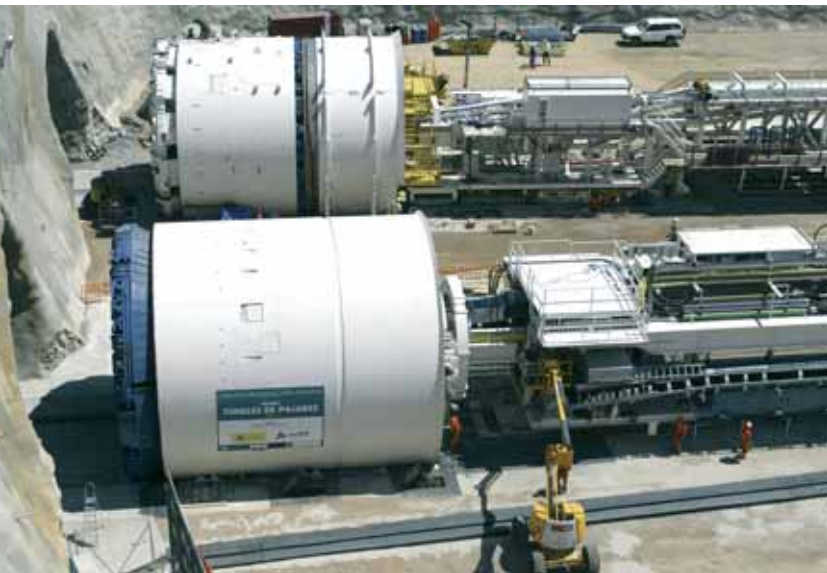
Pajares tunnel. Pola de Gordón-Folledo on the new León-Gijón high-speed train
