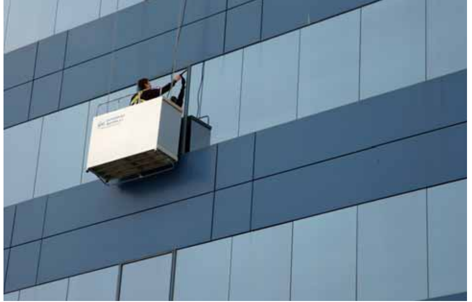
Maintenance and cleaning at the BOE building. Madrid
