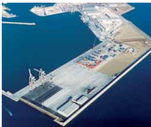
Solid bulk goods terminal and south dock at the port of Castellón
