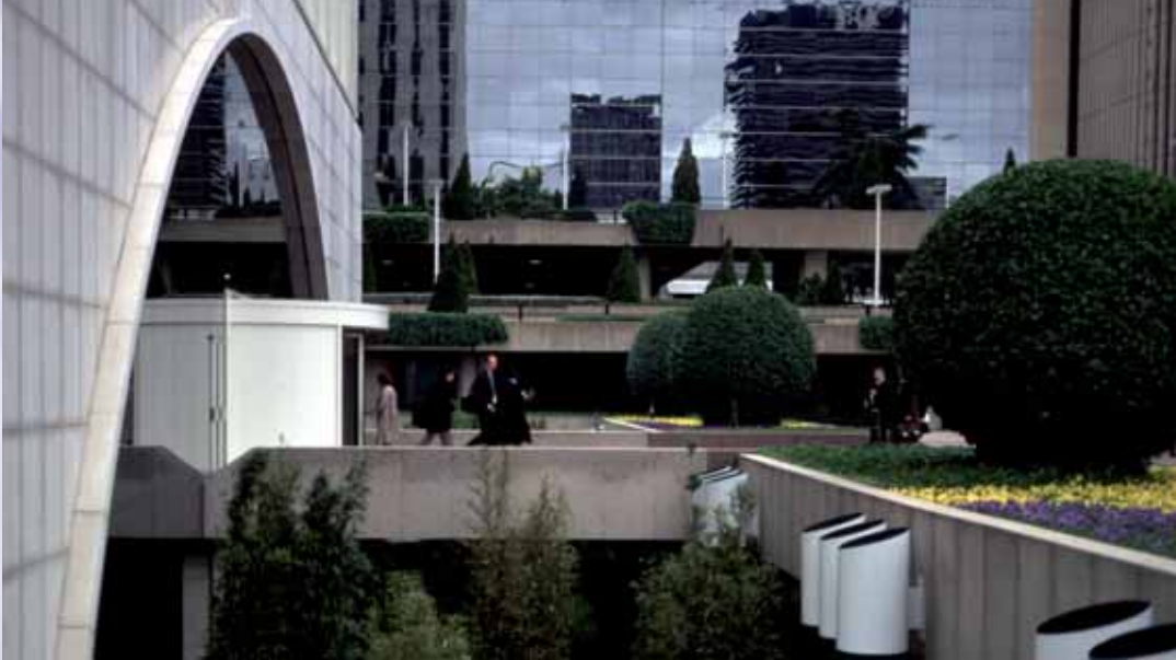
Torre Picaso. Main entrance
