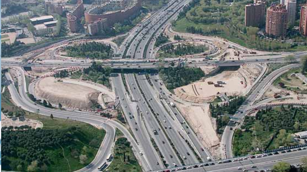
Remodelling work on the junction between M-23-O'Donnell and the M-30. Madrid
