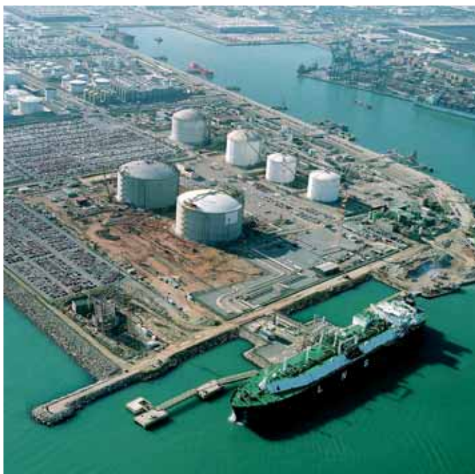
Fifth liquid natural gas storage tank at the port of Barcelona
