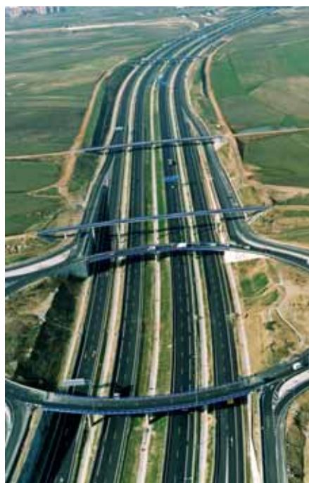
M-50 Dual carriageway ringing Madrid
