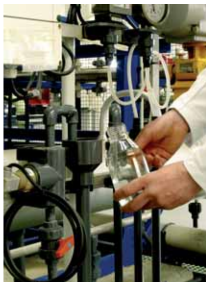
Seawater desalination plant in Tordera. Girona
