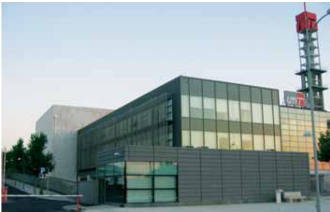
Building for the Castilla-La Mancha television broadcasting company. Toledo
