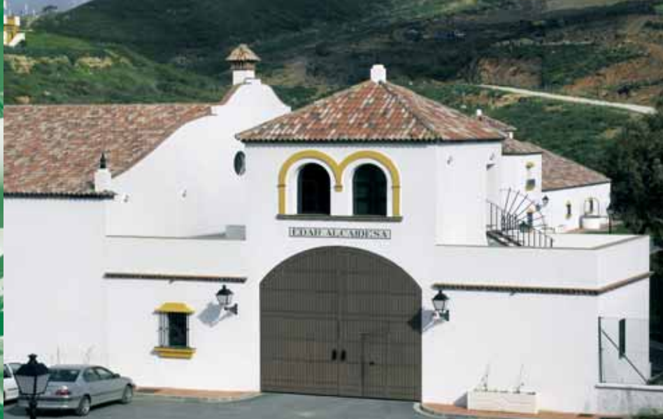
La Alcaidesa wastewater treatment plant. Cádiz
